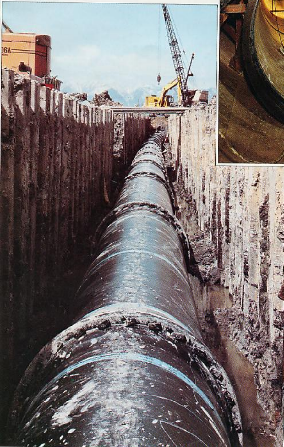
Pipeline using K-Type 1,350mm dia. pipes for on soft ground
