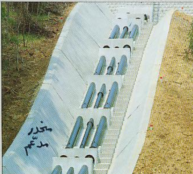
Industrial water pipeline (Polyethylene sleeving method)
