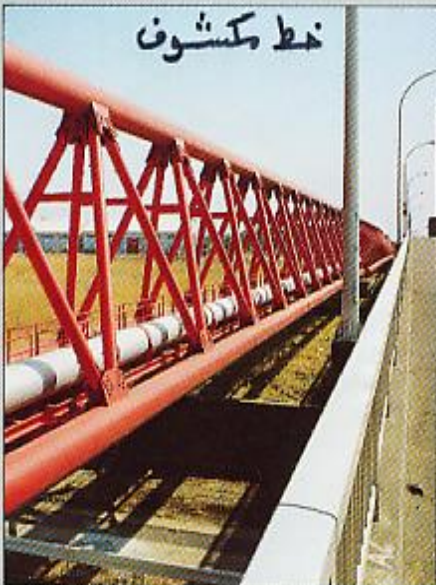
Water supply pipeline (Water-bridge piping)
