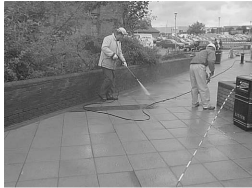
FIGURE 10.9 Cleaning and sealing concrete paving flags.
