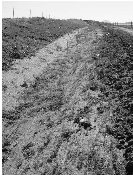
FIGURE 13.2 Synthetic blanket in ditch.
