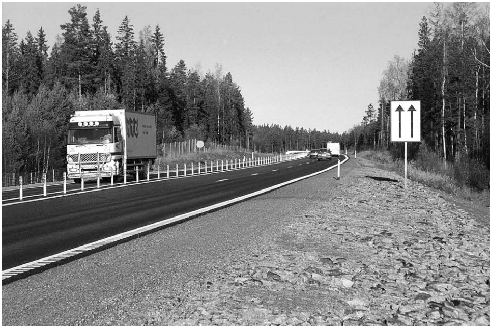
FIGURE 4.1 A Swedish “2 + 1” rural arterial, divided by flexible barrier (Source: Larsson et al., 2003).
