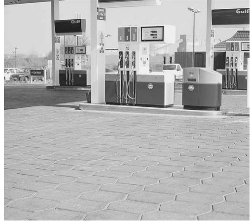
FIGURE 10.3 Segmental paving used to resist petroleum spillages.
