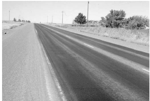
FIGURE 8.10 Bleeding or flushing.
