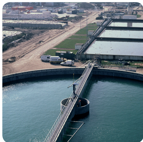
The Tougas wastewater treatment plant.
