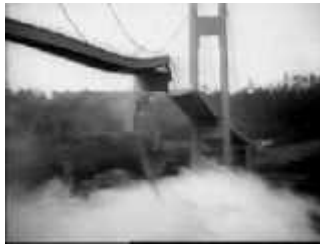
Tacoma Narrows Bridge, Washington, USA.
