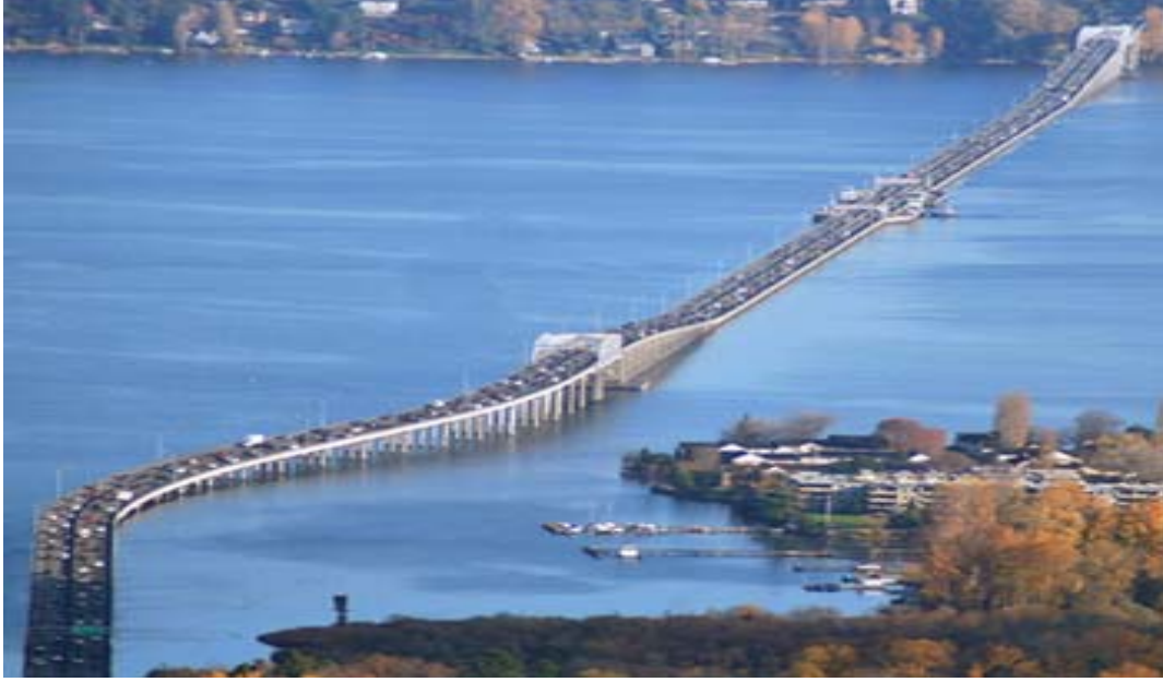
Evergreen Point Floating Bridge, Seattle, USA.
