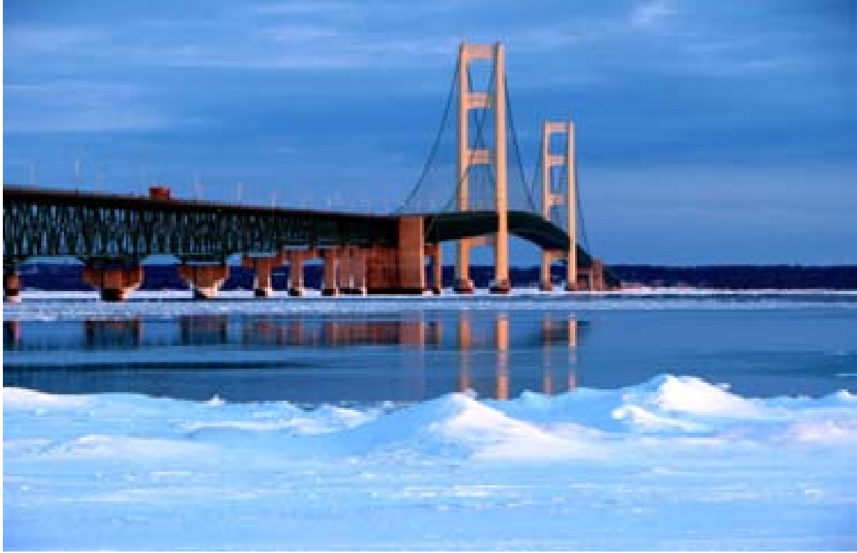
Mackinac Bridge, Michigan, USA.
