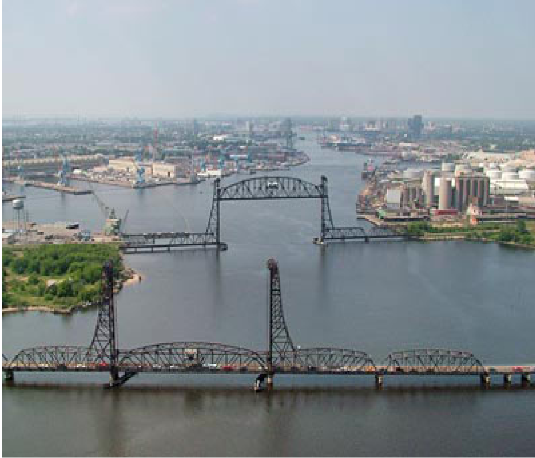
Vertical Lift Bridge.
