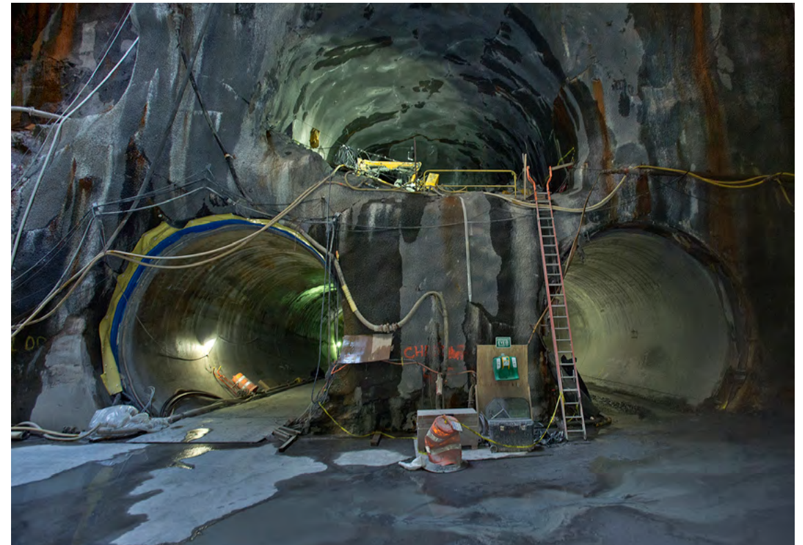
Figure 16: Construction works on Second Avenue Subway
