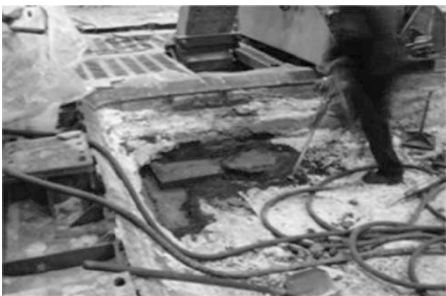
Figure 6. Bottom patching
