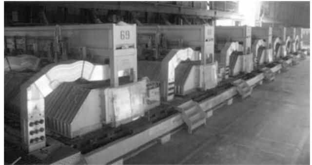
Figure 8: Completed Seven D18+ Test Cell.
