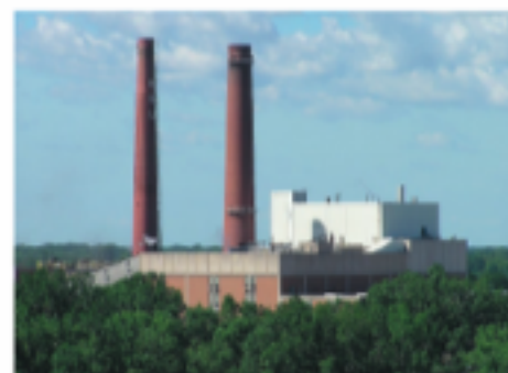
FIGURE 1.19 A coal-fired power plant at Michigan State University that incorporates an electrostatic precipitator to remove particulates from its emissions.
