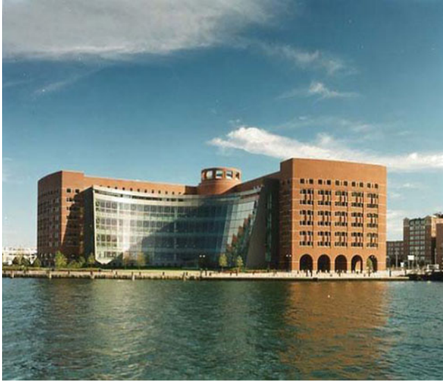
Fig. 23.5 John Joseph Moakley United States Courthouse, Boston, Massachusetts. Architect: Harry Cobb, 1998. Photograph Copyright: Steve Rosenthal, 1998. Photograph reproduced with the permission of the photographer
