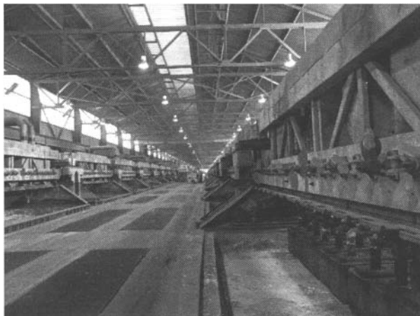
Figure 1: Preparation of the metal surface in Potline 1.
