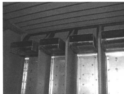
Figure 4. SHEs mounted using a simple one-piece hanger in central inter-cradle space of the demonstration model
