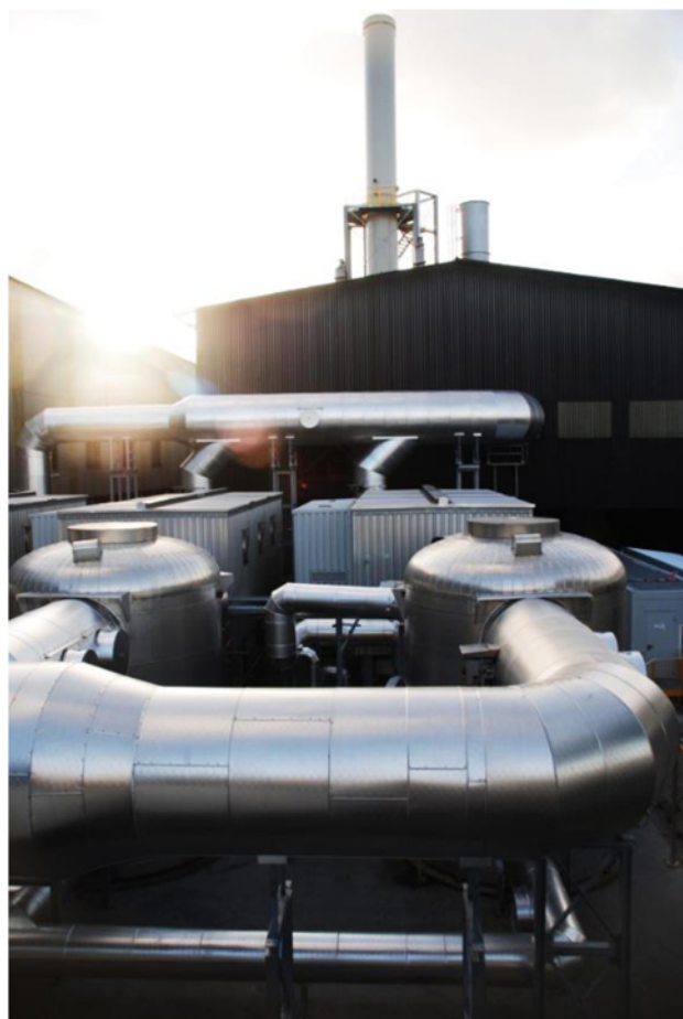
Figure 7: FTS after completion
