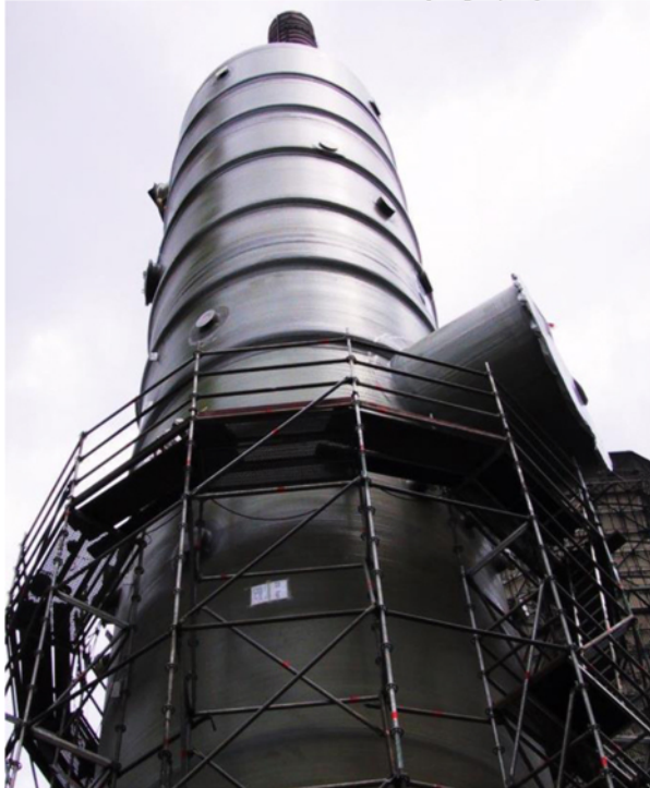
Figure 4: Scrubber system during erection
