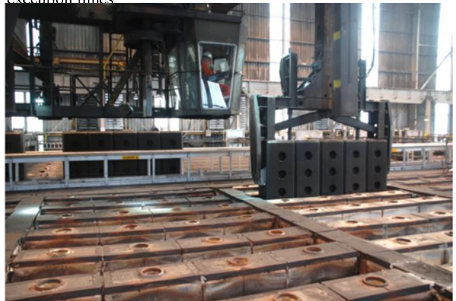
Figure 6: Loading of the baking furnace with the first anodes
