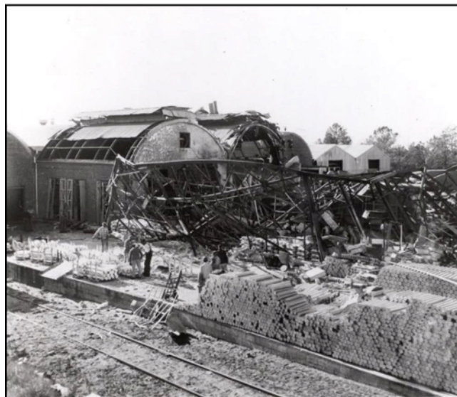
Figure 1 William L. Bonnell Company, Newnan, Georgia explosion of December 27, 1956 which was heard 15 miles away resulted in two workers killed, windows broken in residences, and tops of pine trees broken more than ½ mile away.
