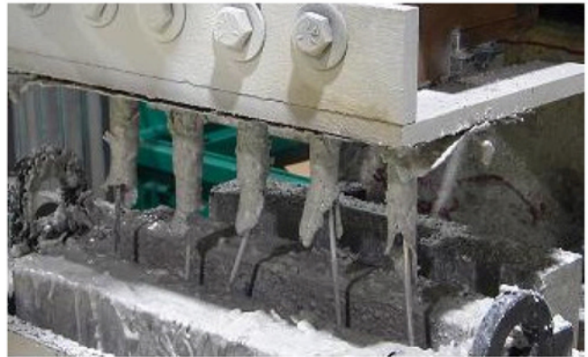
Fig. 5: The consumable guides and the electrode wires Welding
