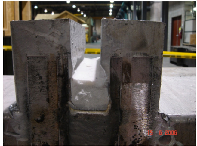
Figure 8: ESW welding system – view from the top showing the slag in fusion
