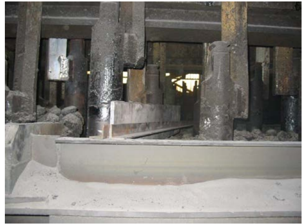
Figure 8. Steel guides were used to vertically support the aluminum plates in VS Soderberg anodes.
