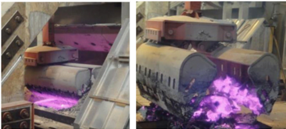
Figure 6: Two snap shots of PTM (pacman) cleaning the anode cavity replacing manual work (Procedure II)
