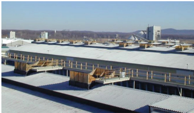
Figure 2. Roofline wet scrubber module exhausts.
