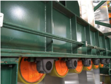
Figure 8. A detail of the framework on the Coil Coating Line.
