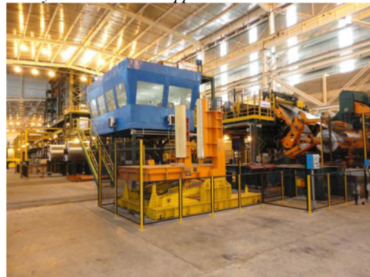
Figure 7. Exit section of the Coil Coating Line.
