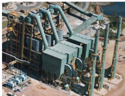
Figure 1: 3 x 4500TPD GSC Units & Bag Filters
