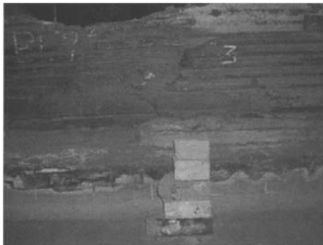
Figure 5. Dislocation of bottom lining up to 117mm.
