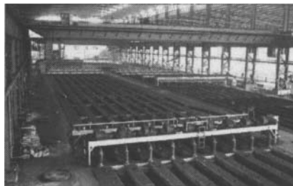
Fig.6 Aohai Carbon's energy saving baking furnace
