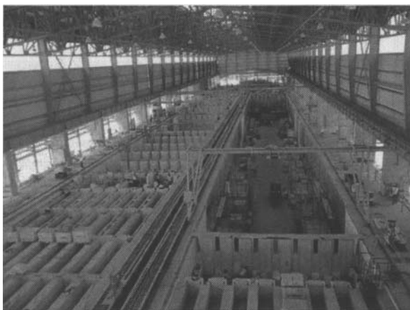
Figure 1: Bake furnace ABF 2 during construction
