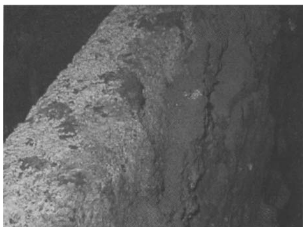
Figure 3. DOE-2 Furnace during a cold cleaning after ~1 year of service.
