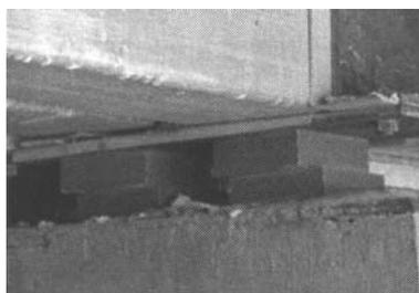
Fig.1. Displacement of insulation bricks under round-end busbars
