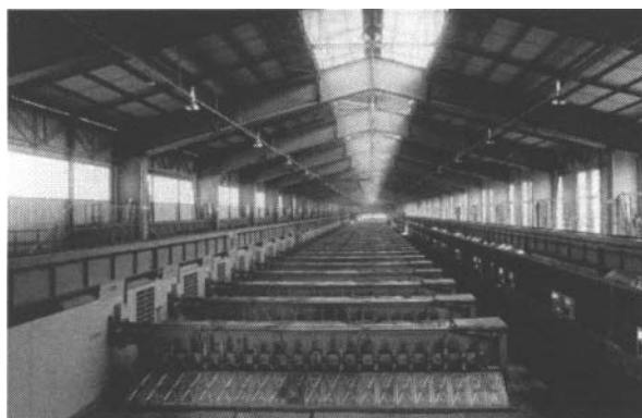
Fig.1: AP30 in operation in G Line at Saint-Jean-de-Maurienne
