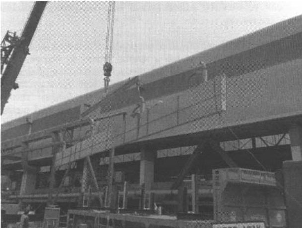
Figure 2. Lifting and erection of distribution airslide
