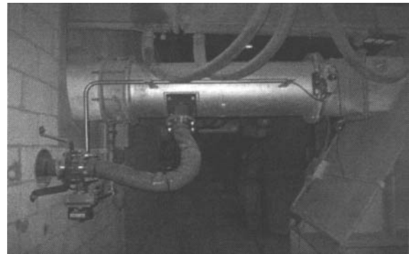
Figure 4. Air injection nozzle and rotating orifice plate at Aluminum Dunkerque
