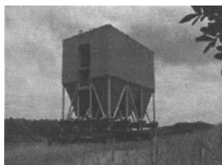
Figure 1b. Fabric Filter – Yarwun Refinery
