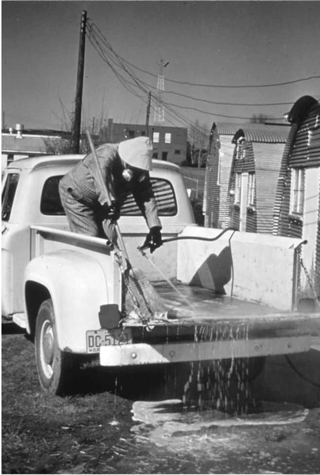
Figure 6.26 Decontamination of truck after spill.
