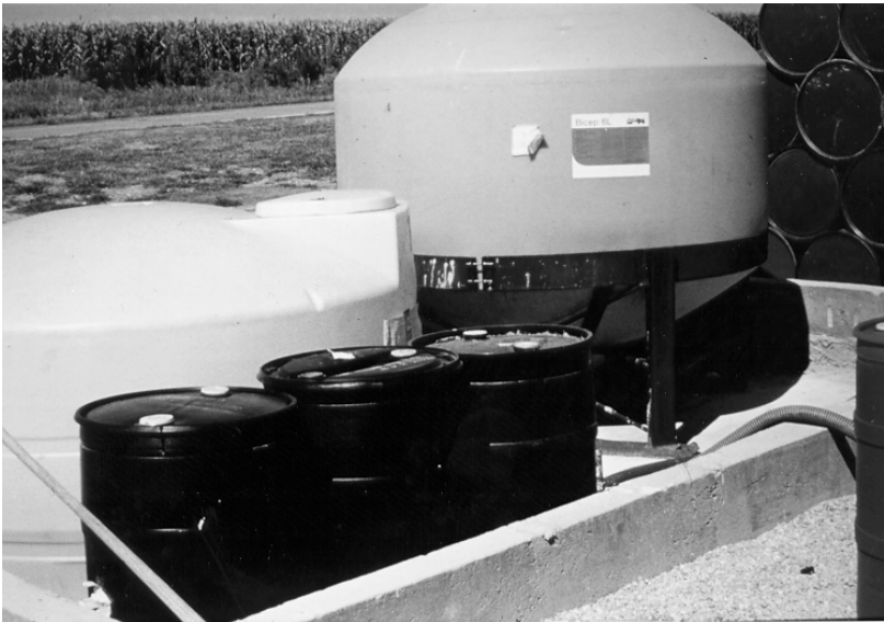
Figure 6.20 Pesticide storage containment. Chemicals are surrounded by a cement curb to contain any spilled material (courtesy of University of Wisconsin-Extension).
