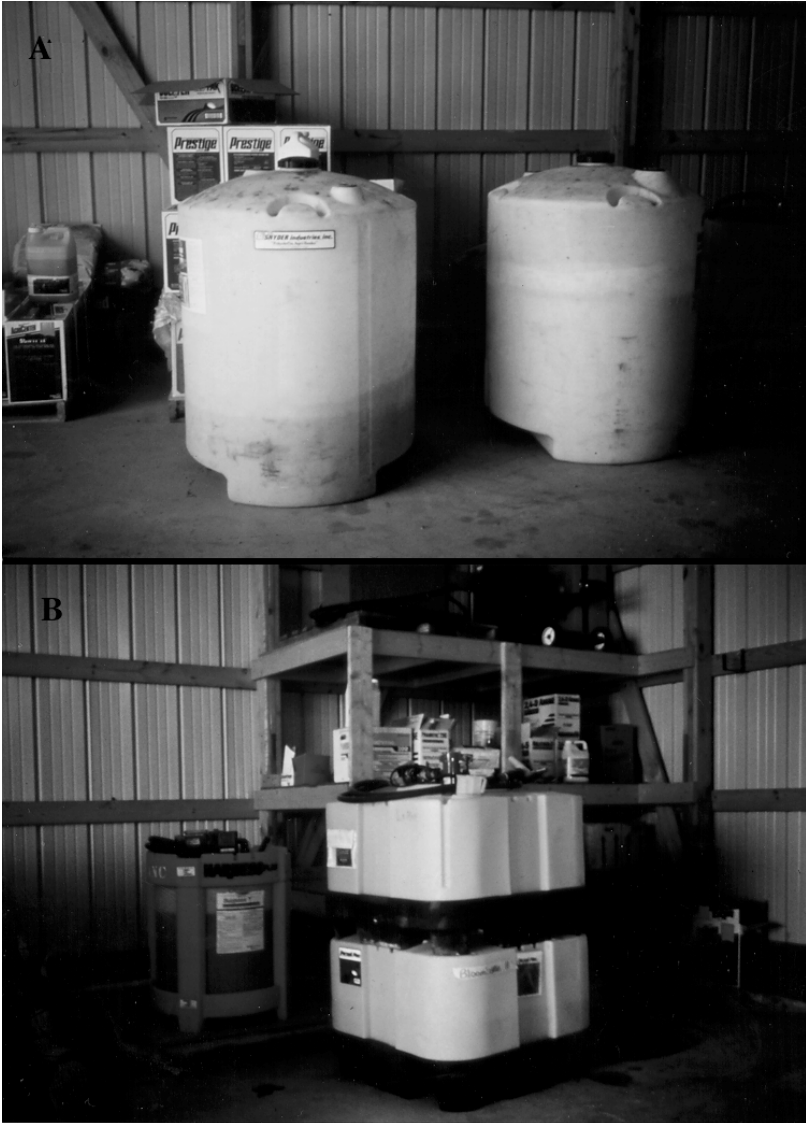
Figure 6.22 Bulk storage facilities (courtesy of Growmark).
