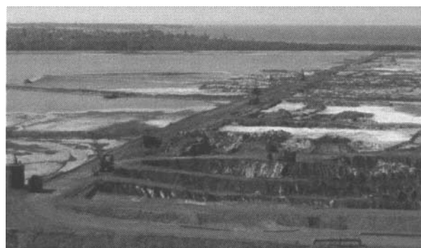
Figure 1. Arrangement of red mud drying and loading at Nikolaev Alumina refinery (Ukraine).
