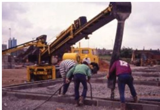
Figure 9.7 Pile caps and ground beams.
