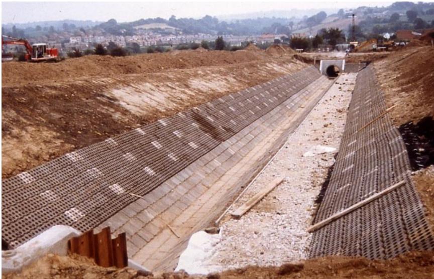
Figure 7.20 Lined vee ditches.
