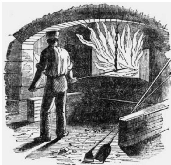
Figure 16.2 Red lead manufacture in the nineteenth century. Courtesy of Elsevier [8].
