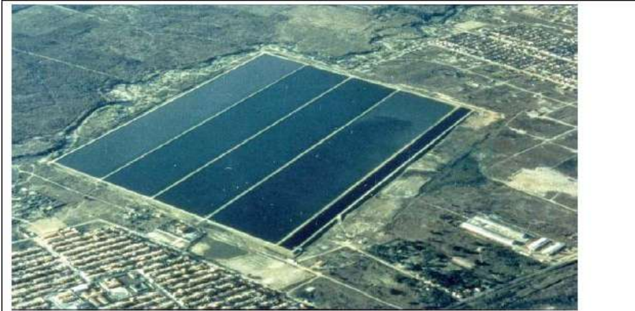
Figure 3. WSP system at Fortaleza in northeast Brazil comprising an anaerobic, a facultative and three maturation ponds (Influent flow 10,000 m 3 /day). Around half the flow is from local textile factories.
