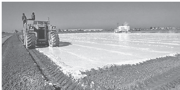
After applying lime slurry to prepared soil, the machine is run in reverse to ensure thorough mixing to the specified depth.
