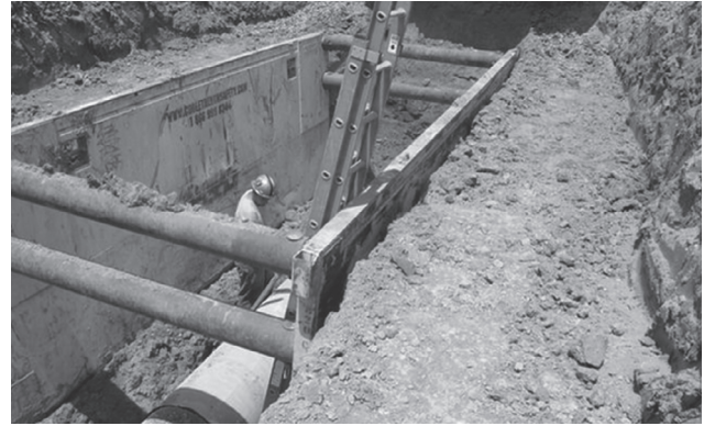
Figure 21.69 Much safer when protected by a trench box. (Courtesy of www.cobletrenchsafety.com/jobprofile.php?id=95 )
