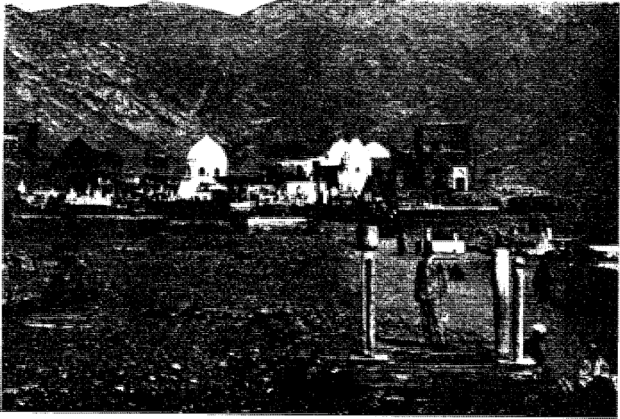
31. The Maalla showing the domes of El Sayyida Khadijah, El Sayyida Amnah, and the ancestors of the Prophet, Abdel-Mottalib and Abd Manaf.
