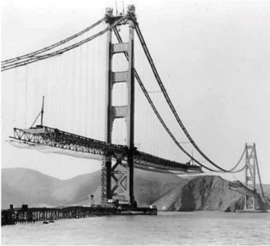
Figure 6.15 Bridge construction analogy. Building up complex, long-range structure in 3D space is often best achieved using repetitive segments assembled in sequence. In effect this is the layer engineering principle, seen here during assembly of the Golden Gate Bridge, where decking segments (some identical, some different) are slung into position to be joined in a pre-determined sequence.
