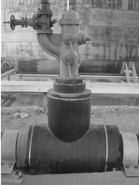
Intact fire hydrant
