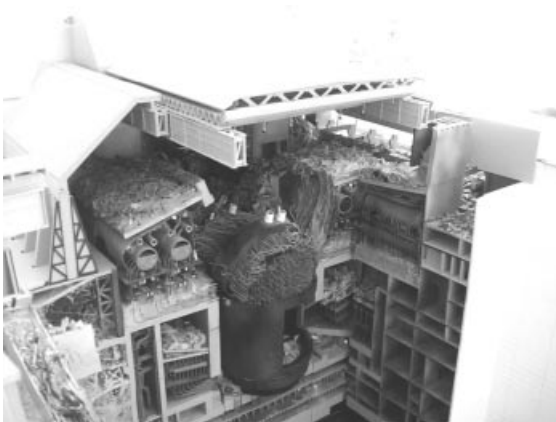
Figure 26.2 Model of the inside of the Chernobyl nuclear power plant after the disaster ( http://en.wikipedia.org/wiki/File:Chernobyl_model.jpg ).
