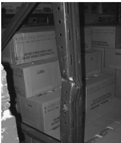
Figure 14.7 Rack support damaged by a lift truck.
