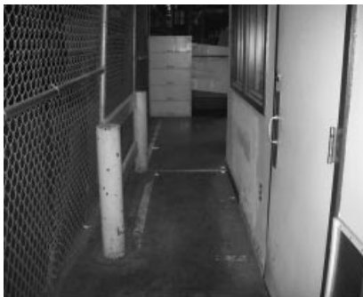
Figure 14.1 Physical barrier to protect pedestrians.
