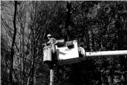
Figure 7.5 Electric linemen may work on electrically energized or de-energized power lines.
