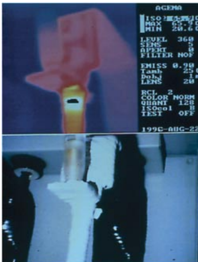
Figure 6.4 Thermograph survey (electrical connection).
