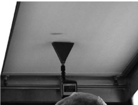
FIGURE 7 Proper scanning of a HEPA filter with a photometer.
