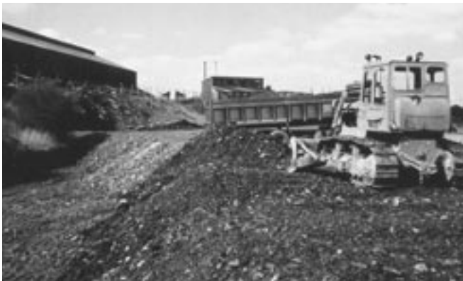
Figure 8.2 Colliery spoil being placed in 2m-deep lifts
