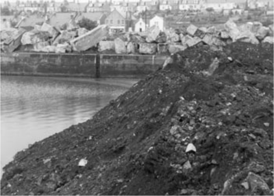
Figure 8.3 Colliery spoil end-tipped into disused dock
