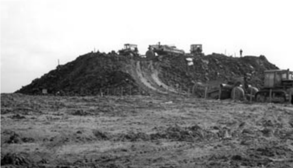
Figure 9.5 Preloading with surcharge of fill
