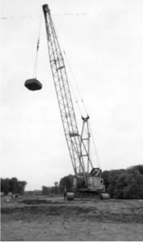
Figure 9.3 Dynamic compaction
