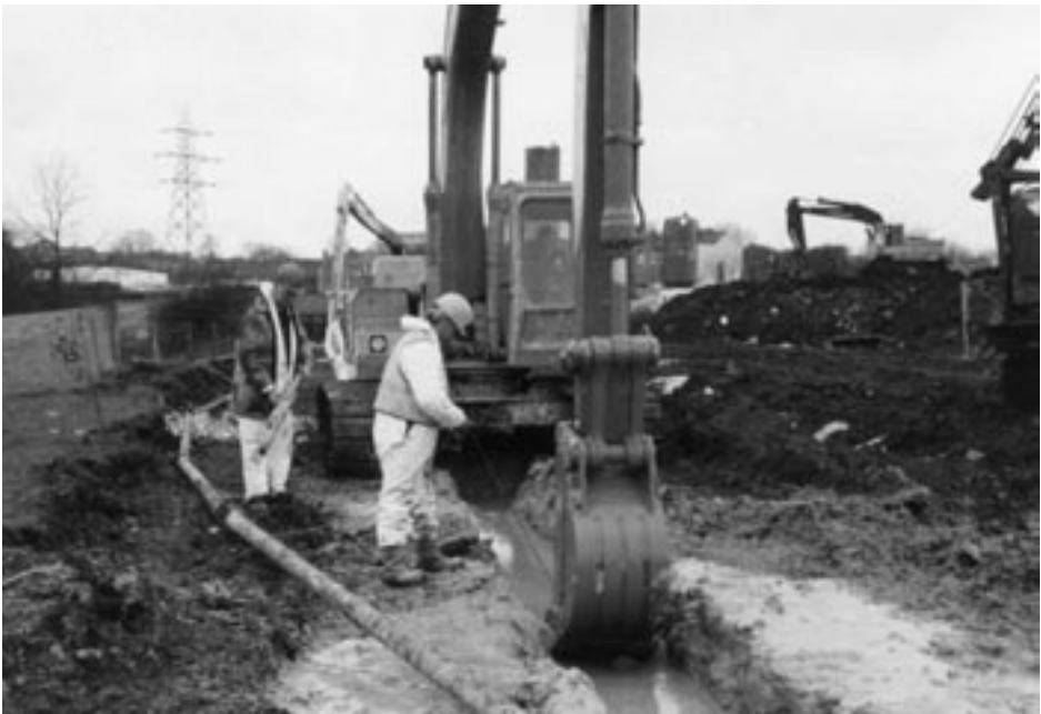
Figure 8.7 Installing a slurry trench cut-off wall
