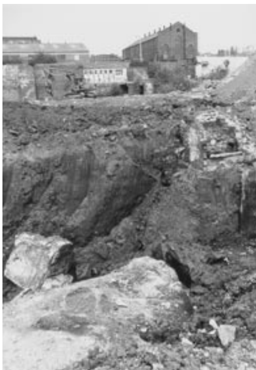
Figure 8.5 Underground obstructions and buried foundations at brownfield site
