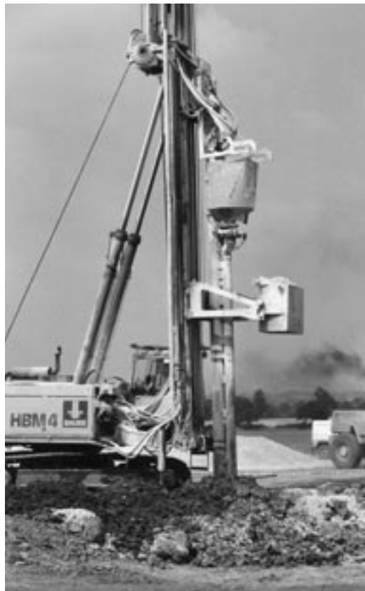
Figure 9.1 Installing vibrated stone column
