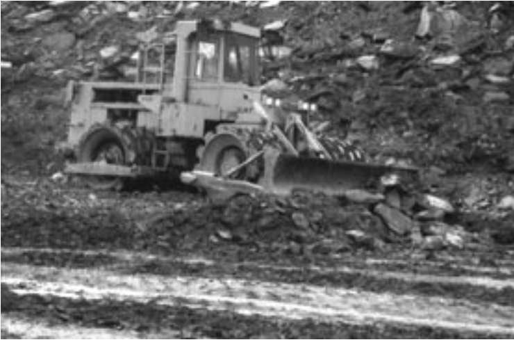
Figure 3.4 Placing an engineered rockfill
