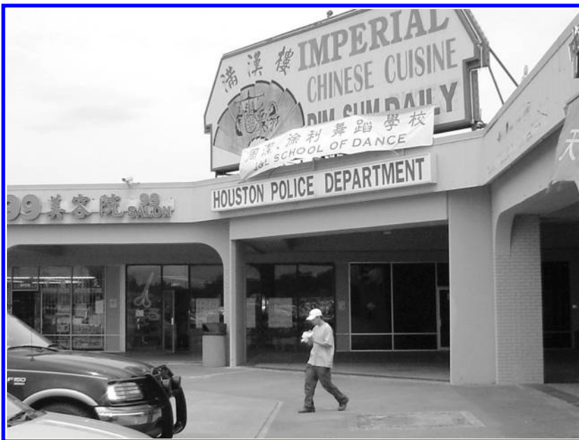
Photo 3-2. A Houston, Texas, Police Department Community Policing Substation located in a shopping center in “China town.” Photo by Cliff Roberson.
