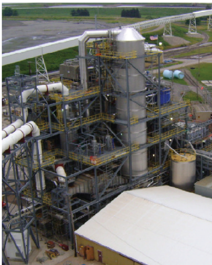
Figure 3. Chilled Ammonia demonstration plant at AEP's Mountaineer power station (Source: AEP).
