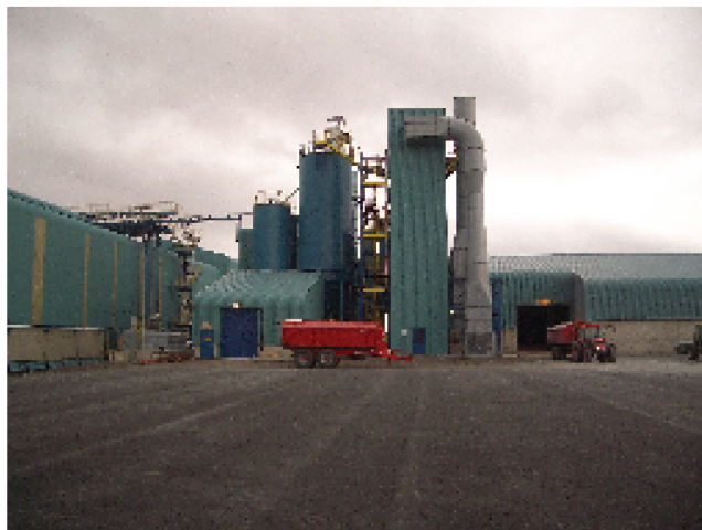
Figure 1. ACM mixing station at Nordural
