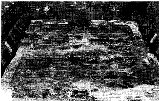
Figure 14. A massive leak of metal into the vermiculite insulation of a cathode has converted its silica content in an aluminothermic reaction and replaced the previous porosity. The material left in the pot shell consist of the former insulation slabs, now reacted and impregnated with 8-10 tonnes of metal. Potlife was 5 days [1].
