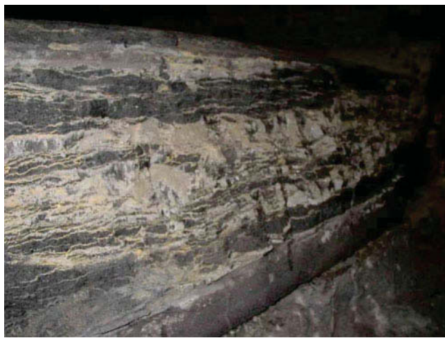
Figure 5: Severely delaminated cathode block, age: 180 days
