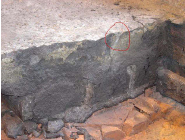
Figure 13. Cracking of end cathode block.
