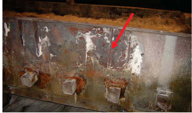
Figure 15: Shell distortion, shown by the arrow, from build up of material on the outside
