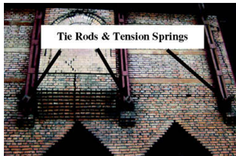
Figure 7: Expansion tie-rods with adjustable tensioning system.
